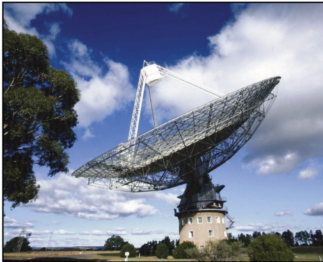
FIGURE 3.2 The Parkes Radio Telescope is located about 400 kilometers west of Sydney, Australia. Radio telescopes are quite different from optical telescopes. Instead of lenses and mirrors to capture visible light, they use a large curved dish and an antenna to view the Universe by receiving radio waves. Viewing the Universe with the radio band of radiation allows us to see phenomena that are invisible to optical telescopes.
